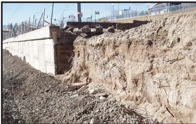
Dismantled MSE Wall, Jan 19
