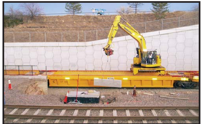
Reconstruction underway, Jan 20
