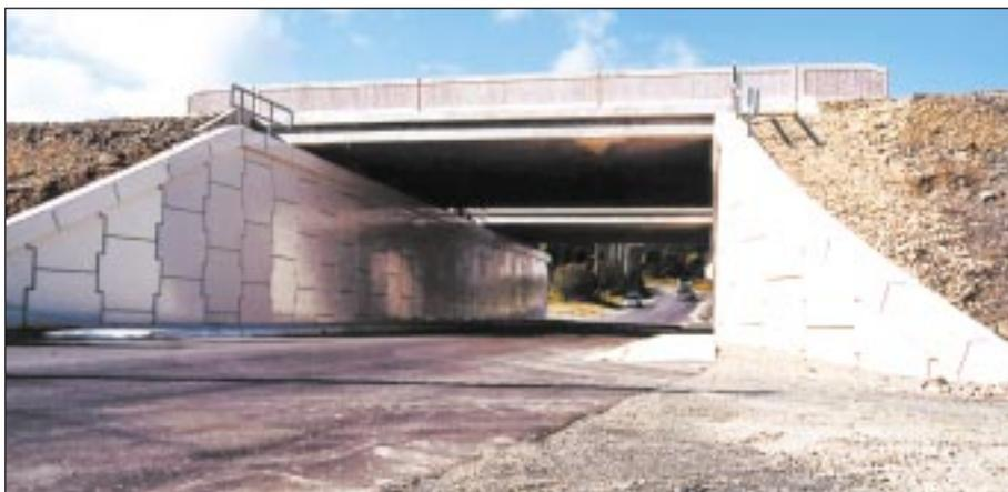
The simple wall alignment makes for an economical and visually pleasing design
