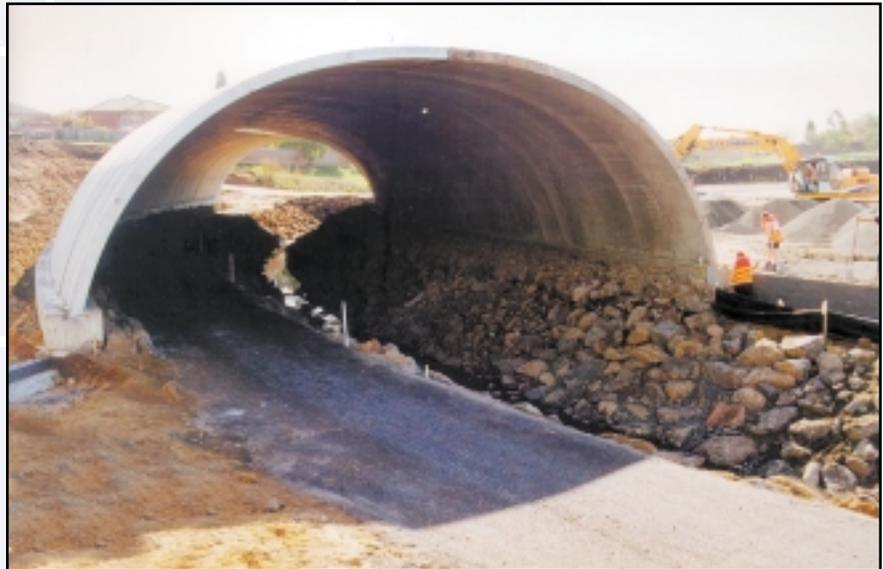
TechSpan was selected for the Edgar Creek stream crossing on the South Eastern Freeway near Melbourne Australia. Reinforced Earth's in house finite element design program was used to custom design the structure. The span is 14.9 m with a height of 4.8 m and length of 54 m. The selected design shape minimized the moments due to loading conditions for the highway and hydraulic loading.
